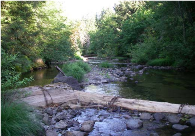
Reach 17 - Unit 850 - Downstream view of habitat structure and reach
