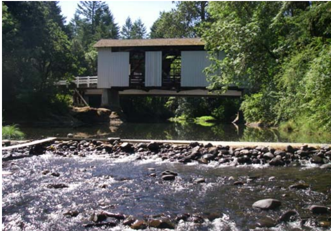
Reach 1 - Unit 53 - Step-over-structure; Stewart Bridge upstream of step
